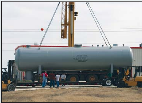
108" Dia. x 45' 0" Horizontal R-134A Receiver
