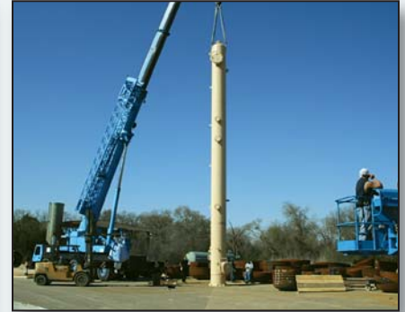
36" Dia. x 52' 0" Vertical Amine Contactor
