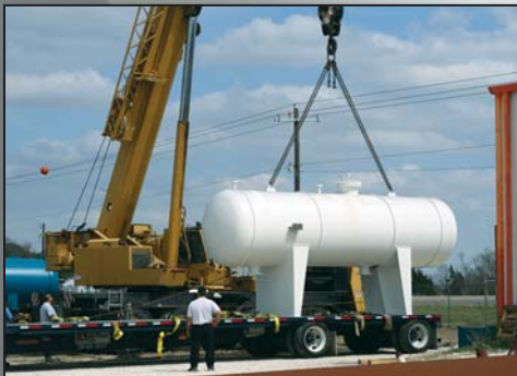
72" Dia. x 24' 0" Horizontal Flash Receiver
